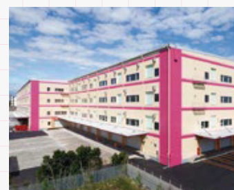
千叶RDC 31,000坪 (102,479m 2 )
