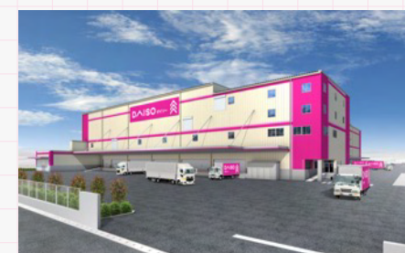
神奈川RDC 8,211坪 (27,145m 2 )
