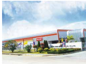
Thailand Warehouse and Factory (101,511 m 2 )
