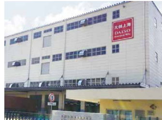
Shanghai Warehouse (33,117 m 2 )
