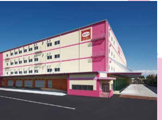
Saitama RDC (59,504 m 2 )
